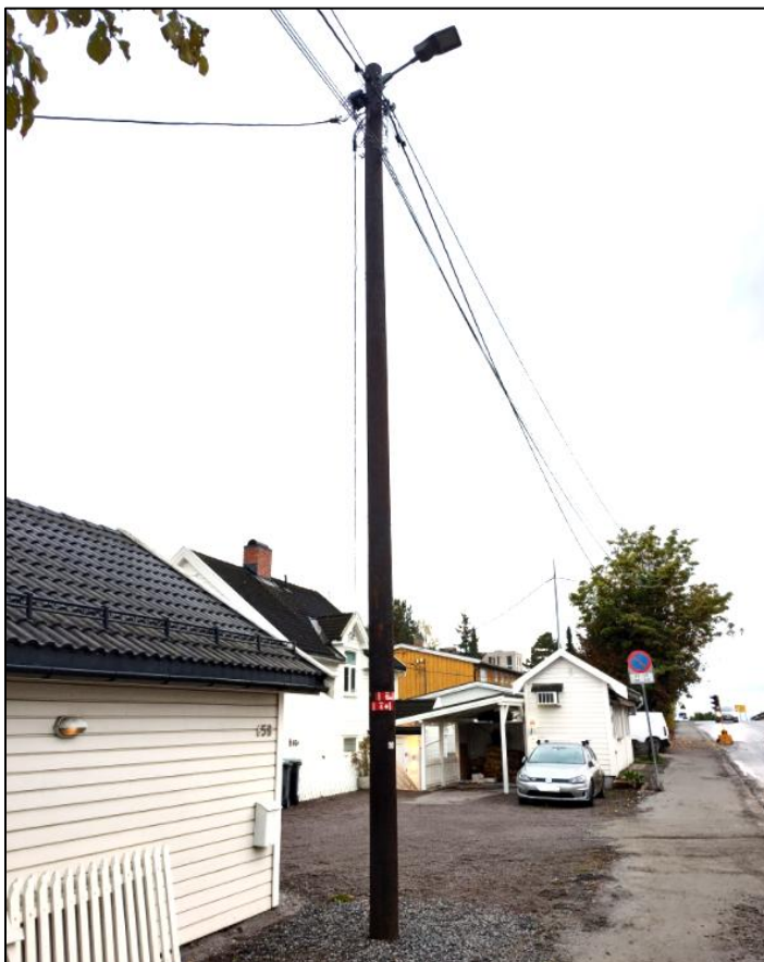
Provisoriske trestolper for strømforsyning.
